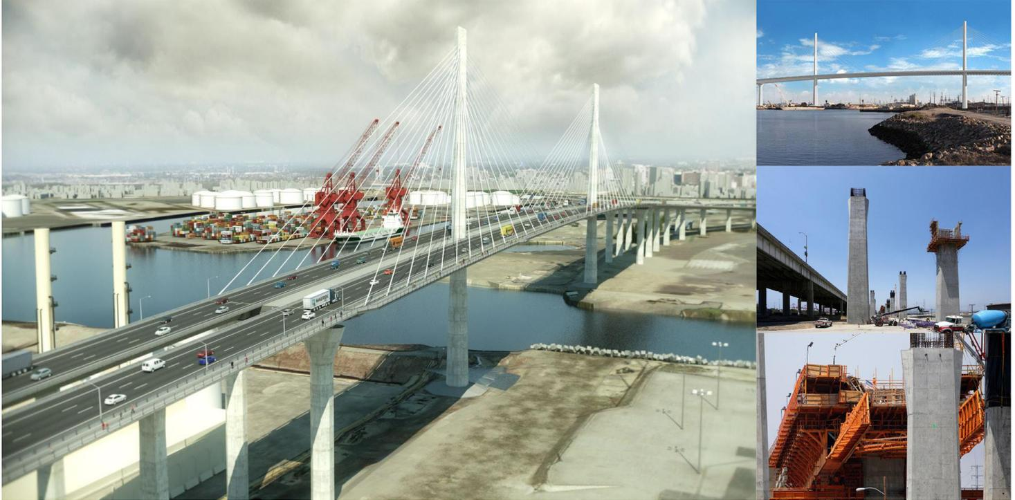
The new Gerald Desmond Bridge is placed in the Port of Long Beach and will replace the existing bridge, with the aim of increasing the vertical clearance over the navigation channel and improve the seismic behaviour.
